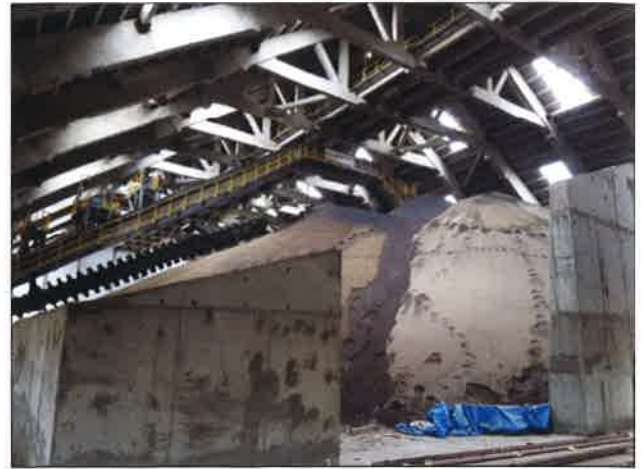
Fig. 4: Photograph of the structure from inside with the material stored
