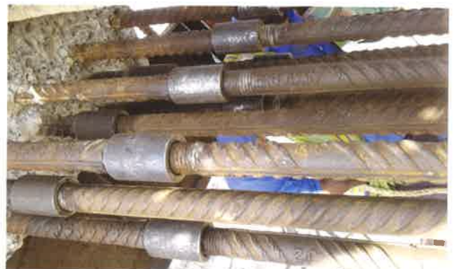
Fig. 8: Mechanical couplers for reinforcement
